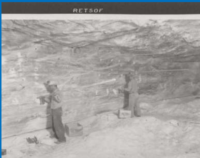
Loading holes with explosives..
