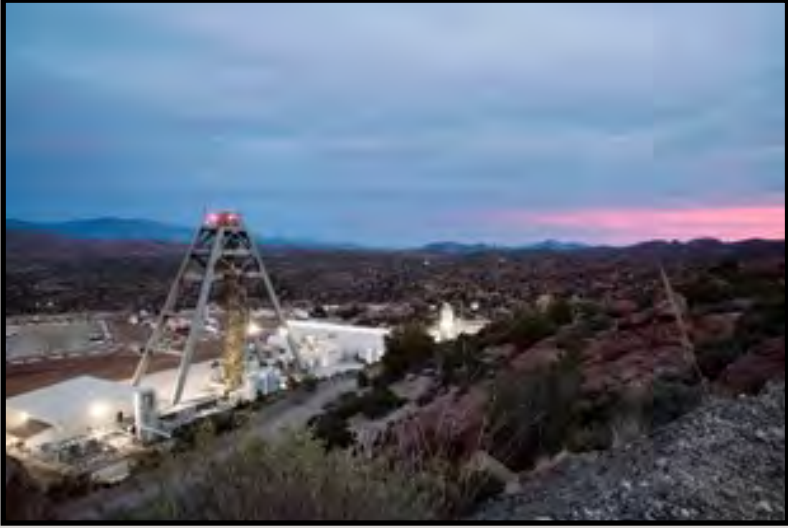
Shaft in the Superior-Resolution copper prospect in Arizona.
